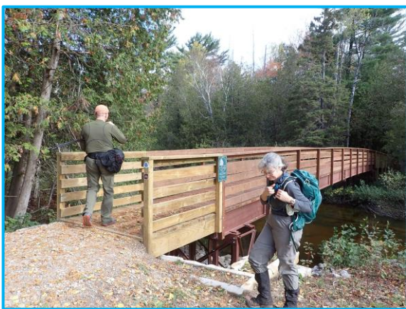
Petoskey Bear River Bridge
