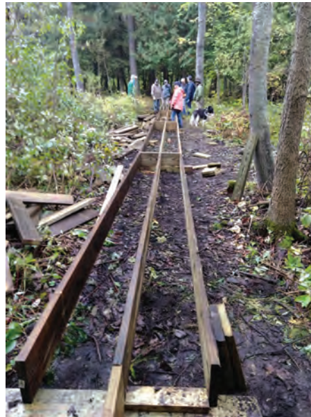
Building puncheon. (L to R): 1st placing sills, 2nd attaching the stringers, and 3rd adding deck boards and curb
