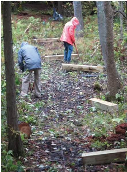
Building puncheon. (L to R): 1st placing sills, 2nd attaching the stringers, and 3rd adding deck boards and curb
