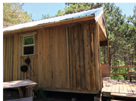
More siding was added to finish this wall
