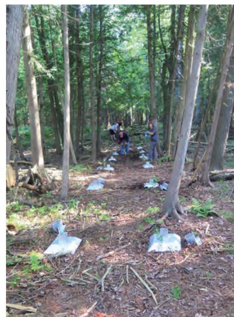
Step 1. Laying out the "swamp pans" for the new boardwalk.
