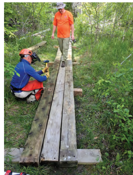
Old beams from the sunken boardwalk were turned into new puncheon
