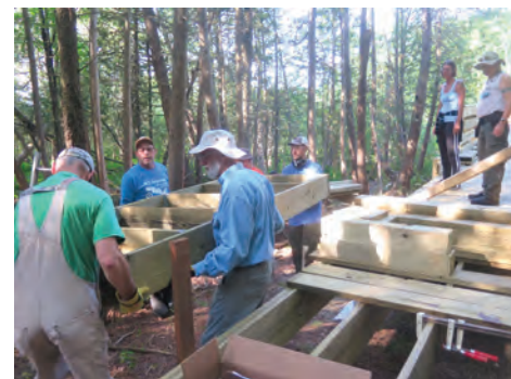
Seven "boxes" were built, 4 feet wide and 10 feet long. These were the base support structure for the boardwalk.
