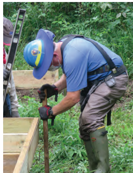
Setting swamp pan on new puncheon bridge
