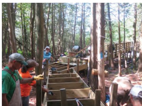
The "boxes" were bolted end-to-end once they were level.
