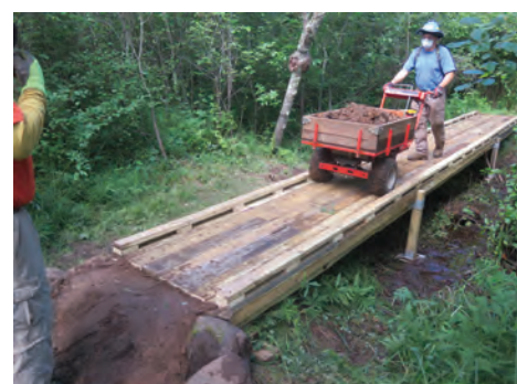
Rock/dirt ramps for new puncheon bridge
