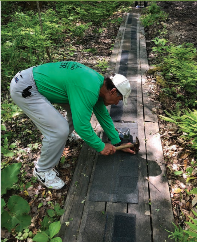
Nailing down shingles to prevent slippery boards when wet. Photo: Shari Sanderson
