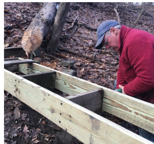
Spacers beneath the deck
