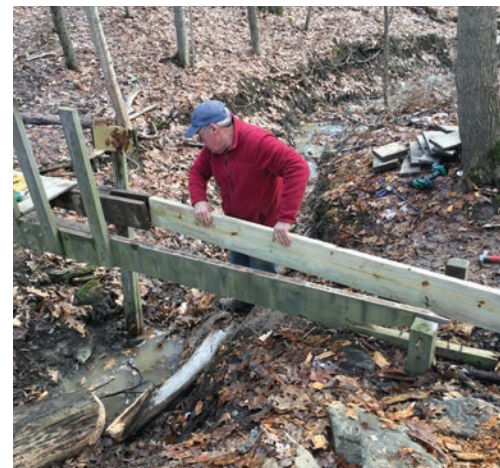
A new segment fits right into the original bridge frame.
