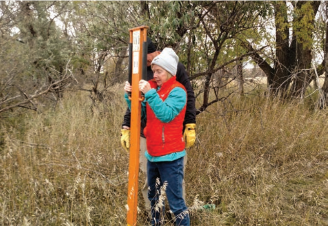
Ginny and Bill Newman pounding in a Carsonite post with a special sign driver. Bill, Ginny, Tom and Mary Moberg spent a weekend at Lonetree improving NCT signage, installing or repairing over 50 needed signs.
