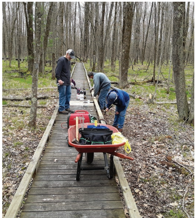
The crew installs replacement boards where needed on this long swamp boardwalk.
