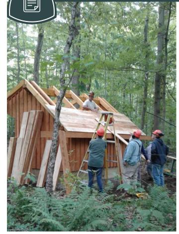
Last summer one of the Symposium shelters was re-built in the woods, near the west end of the Trail in N.Y. These post and beam shelters are much easier to build than the traditional style using whole logs, and safer, too! Photo: Donna Flood
