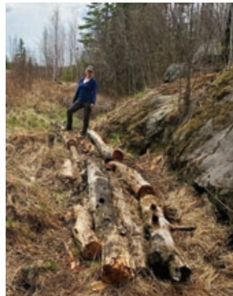
Rachel Jarvis, in the process of laying tree trunk planks on the Trail next to Seahorse Lake.
