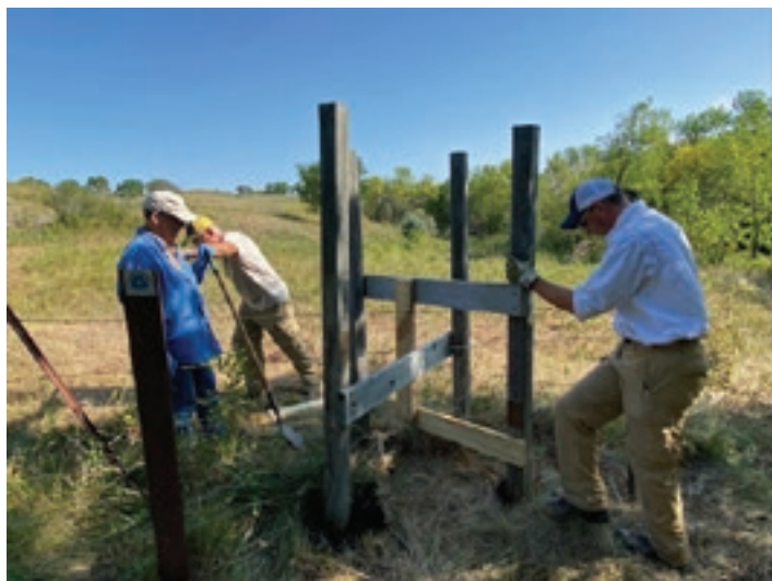
Above: Modifying fence stiles for trail users with shorter legs.
