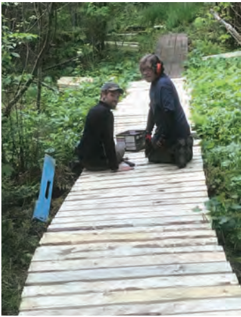
Left: Nailing deck boards to puncheon on National Trails Day 2022, at the Silver Creek project site. Bottom Left: Left to Right: Bob McNamara, Lucy Evashevski, Patricia McNamara, and Tom Walker celebrate the end of a workday on the Naomikong Overlook project. Several crew members camped and worked for a week in September. Photos by Tom Walker
