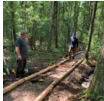
Jack Barnhill (left) and Dan Driesenga work on a turnpike project near Baldwin, MI.
