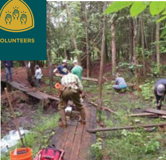
Puncheon project near Russian Creek at North Central Michigan College.
