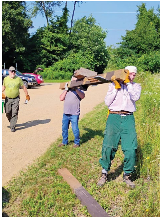
A kiosk is moved in response to a trail reroute.
