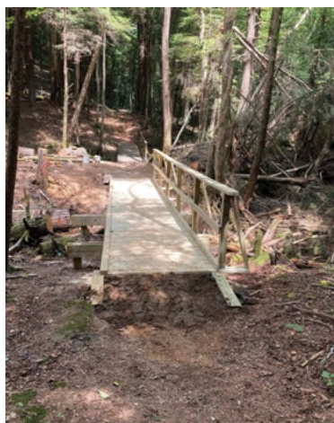
Liggett Bridge, Clarion County, PA
