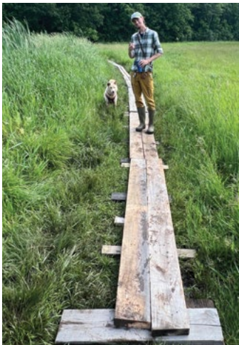
MALT Trails and Volunteer Manager Liam Hickey on newly installed puncheon.
