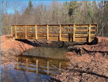
Bush Creek Bridge, Michigan.
