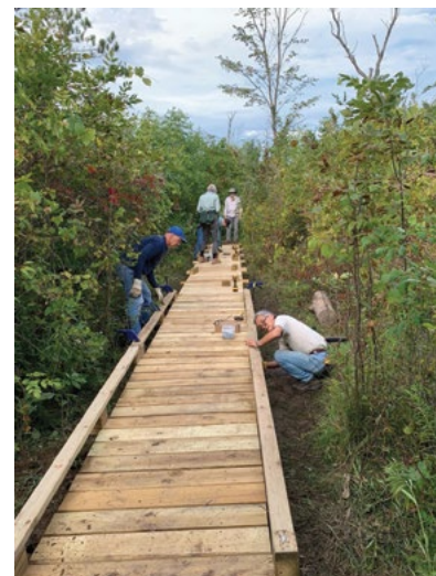
Above: A work crew installing anti-slip treads at Sterling Marsh.
